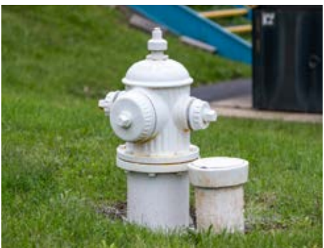
Stripped down fire hydrant before paint is applied
