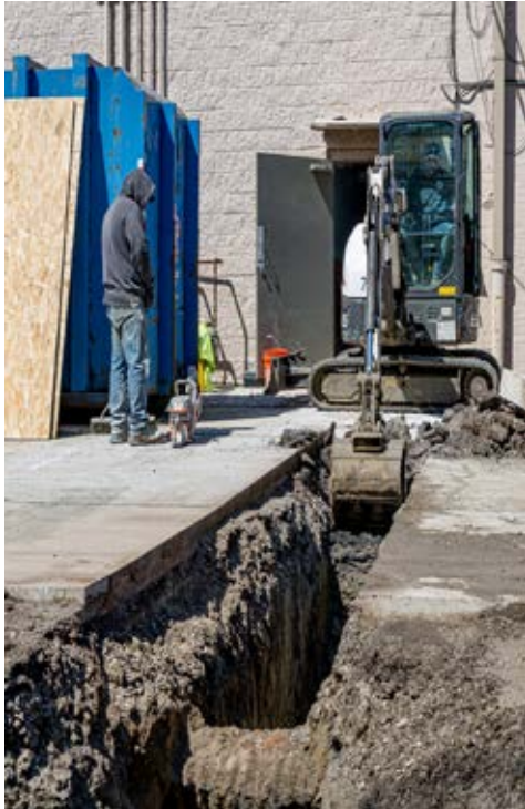
Final lead line removed.
