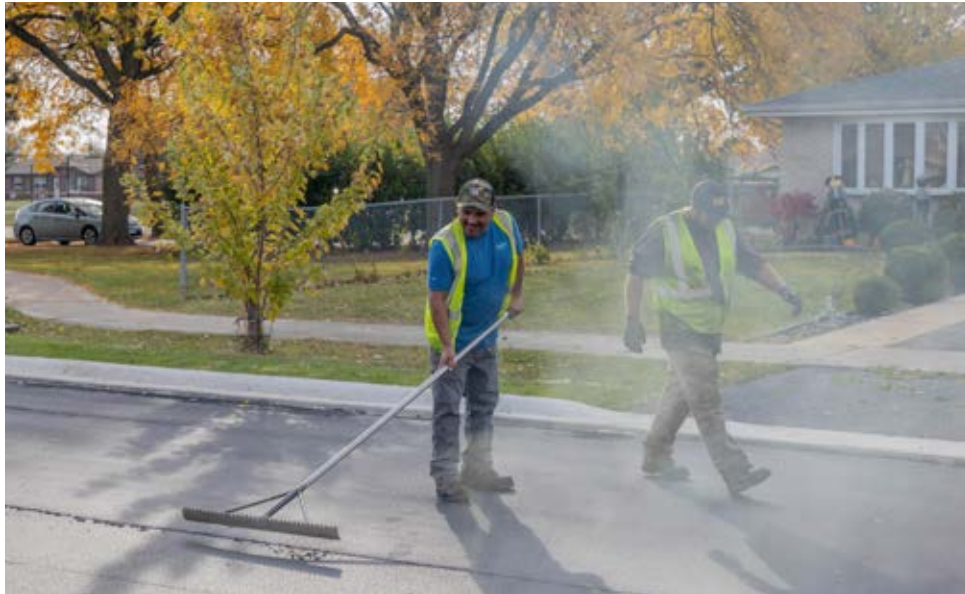
Road workers smooth out a freshly paved road.
