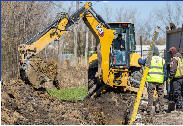
Dirt is removed to access the water line and expand it.
