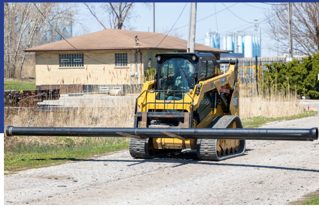
Long pipes are transported to the ditch for connection.
