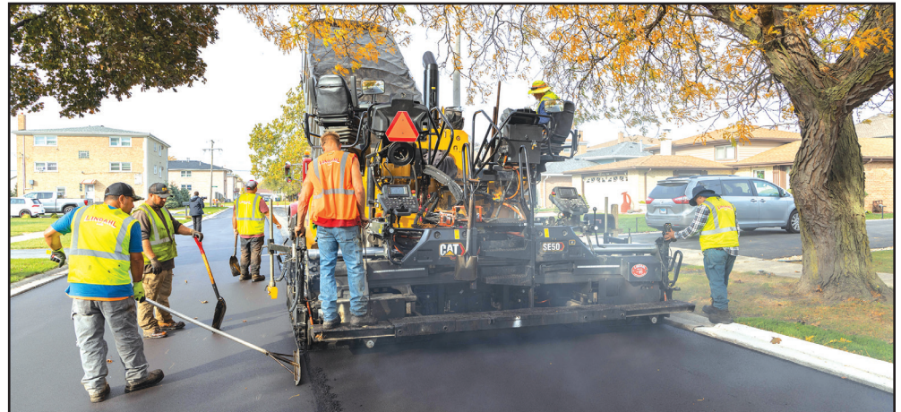
A snapshot of the repaving process in action!
