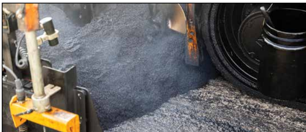
The paver heats and drops asphalt before paving over it.
