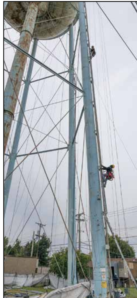
Workers climb the Water Tower for exterior maintenance.
