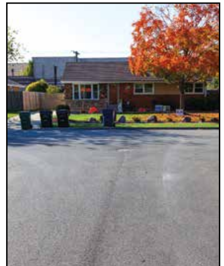
Residents enjoy newly repaved roads.
