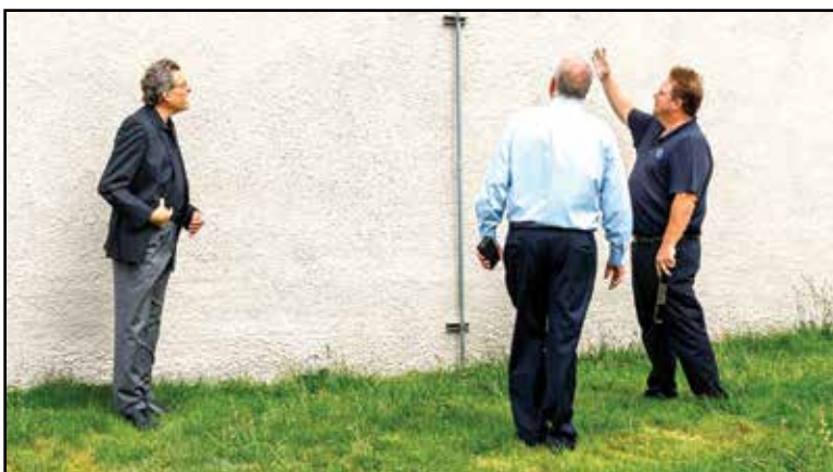
Mayor Landek (left) Trustee Gary Lewis (center) and Water Plant Operator William Green (right) review the above ground tank completed repairs.
