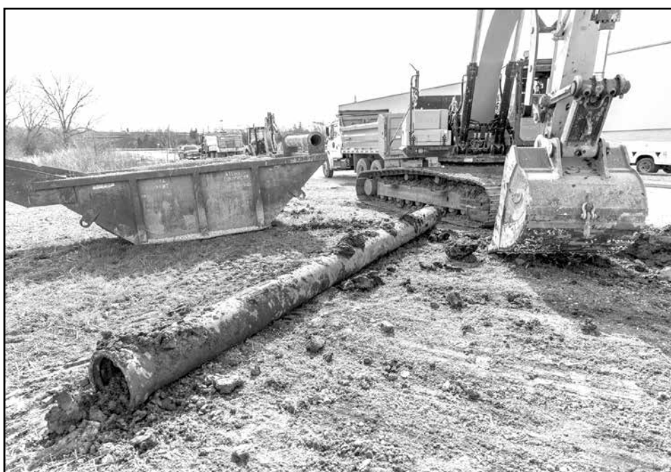
A broken section of a water main.
