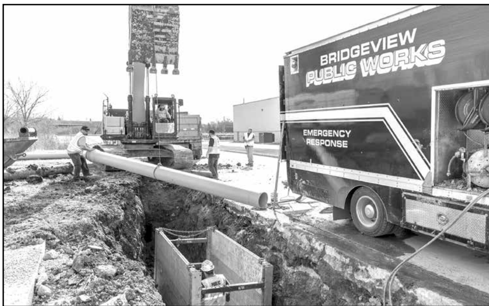
A new pipe gets lowered into the trench.
