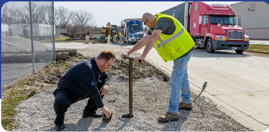
Bridgeview Water Plant Operator William Green (Left) guides Bridgeview Public Works employee John Kramarsky (Right) in placing a valve key into the ground to shut off water on a main break site.
